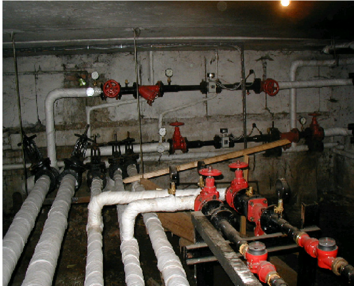
Fig. 28: Pipe insulation, valves, building level heat and water meters installed at a building
